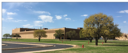
498,810 SF 8600 N. Central Fwy. Wichita Falls, TX
