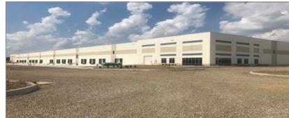
324,000SF 3280 Southpark Plac Grove City, OH
